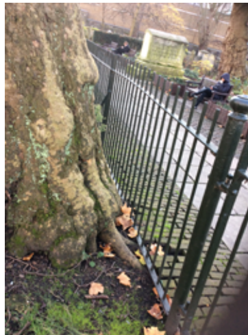
Damage to pavement from buttress roots.
