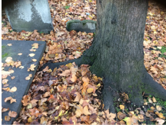
Root spread causing damage to tomb
